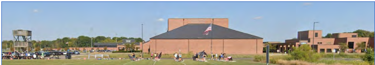
Figure 1: Bradley High School
