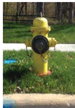
Example of 5" Storz Hydrant
