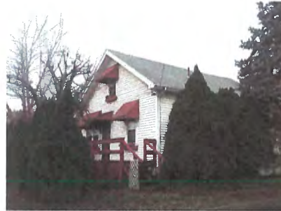
APPARENT ENCROACHMENTS: NONE.
