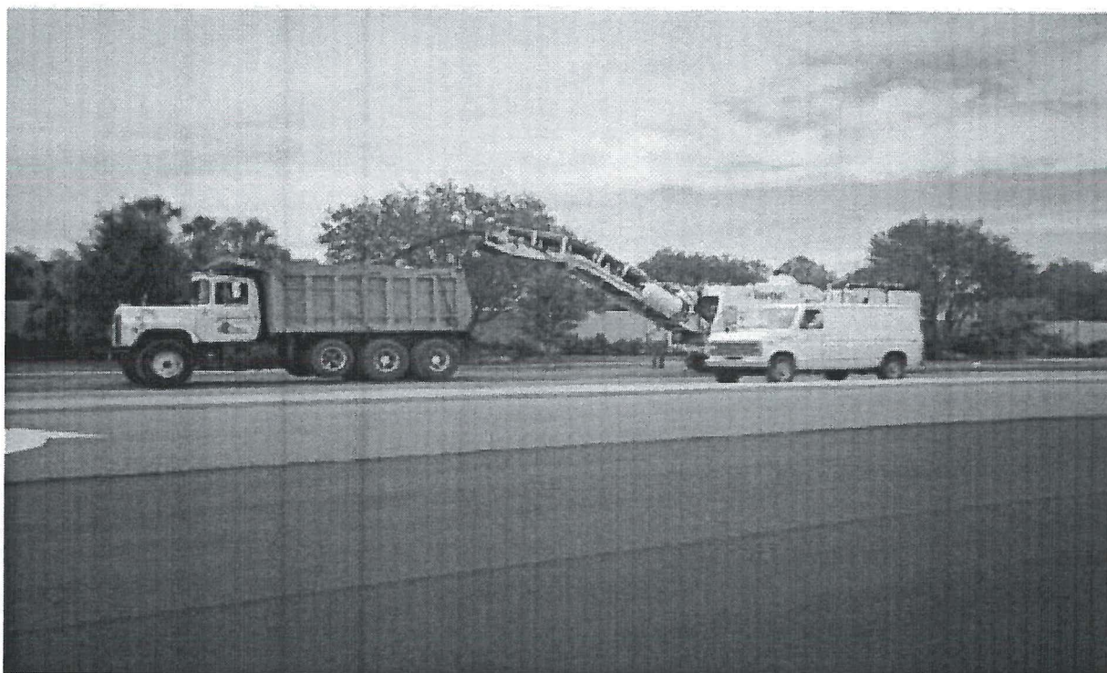
Figure 2.2 Typical Roadway Excavation Process
