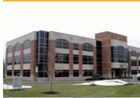
Small and larger office buildings and residences
