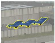
The above image shows a properly placed PV System, highlighted in yellow, in a non-intrusive location atop the historic structure.
